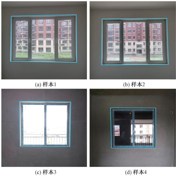
图11 窗框检测可视化结果 Fig.11 Visualization results of window inspection
